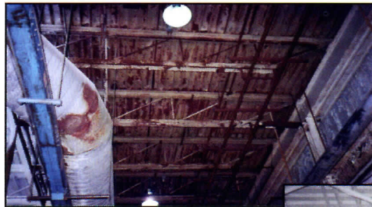
Roof Deck and Joists, before
